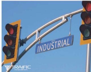
On existing bracket arm for vertical traffic lights
