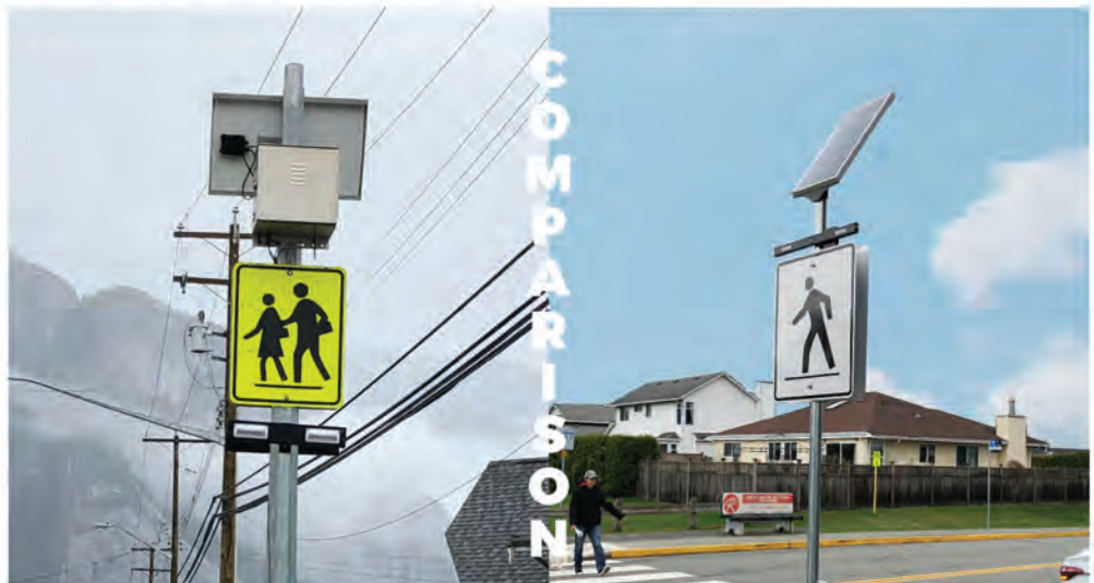
COMMON SOLAR PANEL SYSTEM
