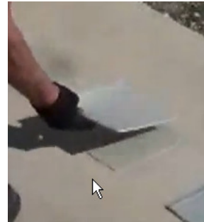
Placing Second Pad
